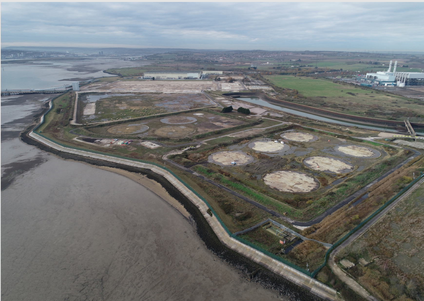
Aerial Photo of the Converter Station Site at Kingsnorth
