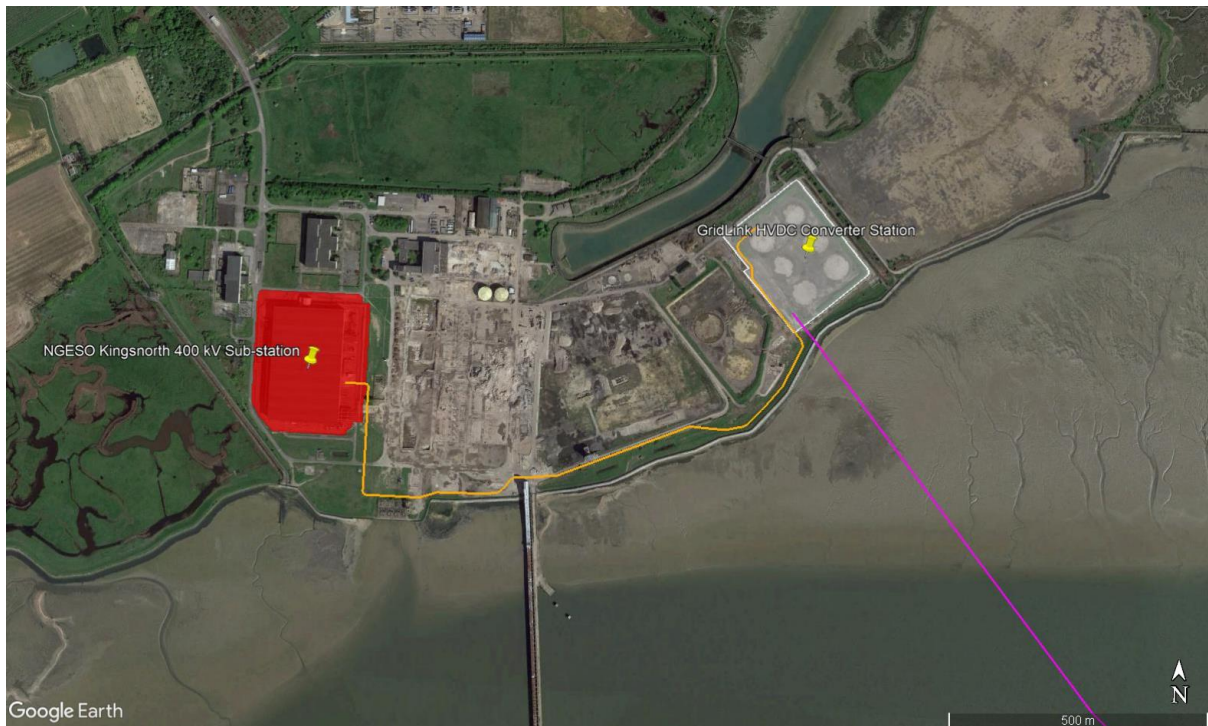
Figure 3: GridLink Converter Station Site and Underground Cable in UK
